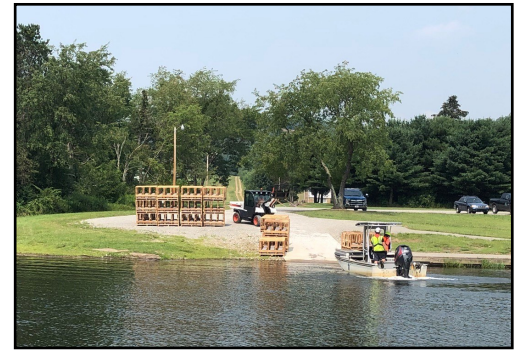
Vertical plank boxes to be installed in Donegal Lake.
