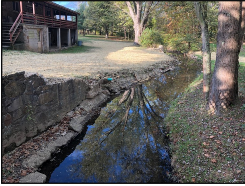
Bank stabilization along an unnamed tributary to Mill Creek.
